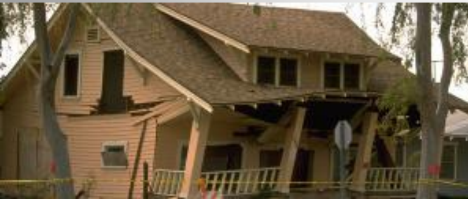
Dwelling in California with Failed Wall Sheathing
